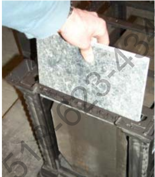
Inserting the Side Stones
