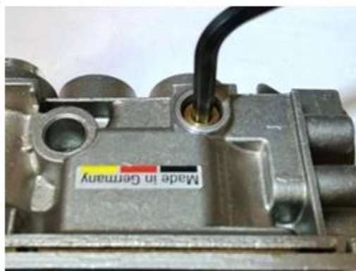
Location of Low Pressure Adjust Screw (Under the fireplace)
