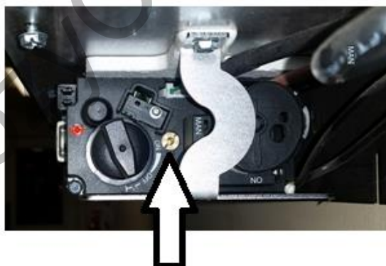
Location of the Fuel Conversion Screw (Under the fireplace)
