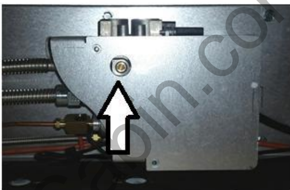
Location of Low Pressure Adjust Screw (Under the fireplace)
