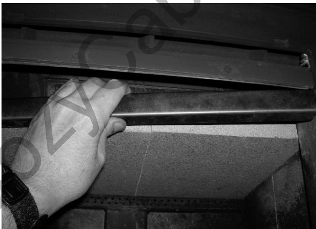
Figure 18 - Removing/Replacing the Baffle for Inspection
