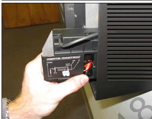
Step 1: Locate Reset Button on Receiver
