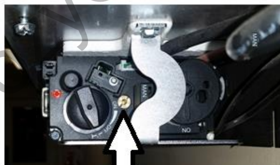
Location of the Fuel Conversion Screw (Under the fireplace)
