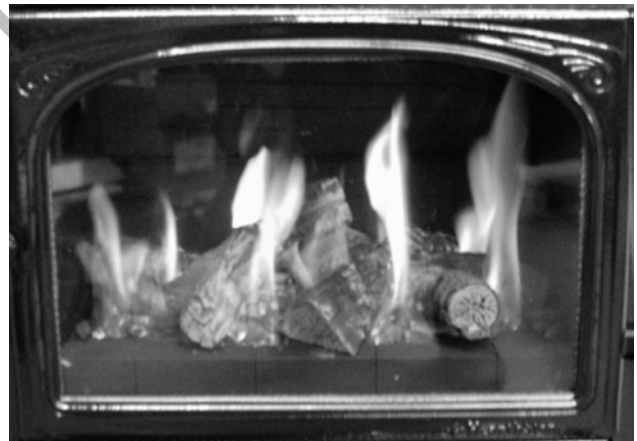
Figure 21 – Typical Burner Flame Appearance
