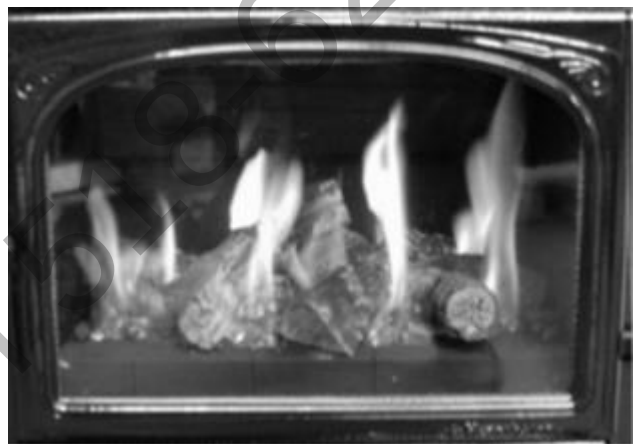
Figure 21 – Typical Burner Flame Appearance
