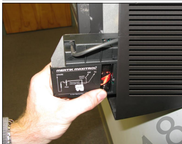
Step 1: Locate Reset Button on Receiver
