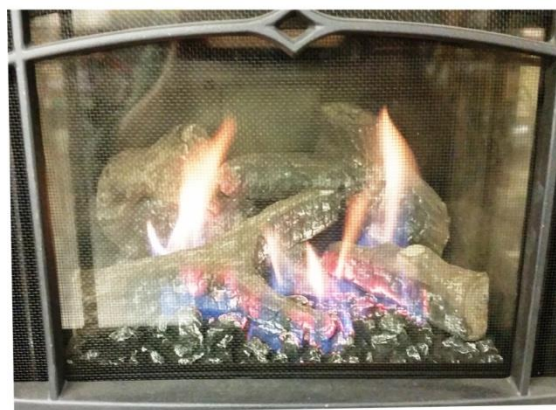
Figure 40 – Typical Burner Flame Appearance
