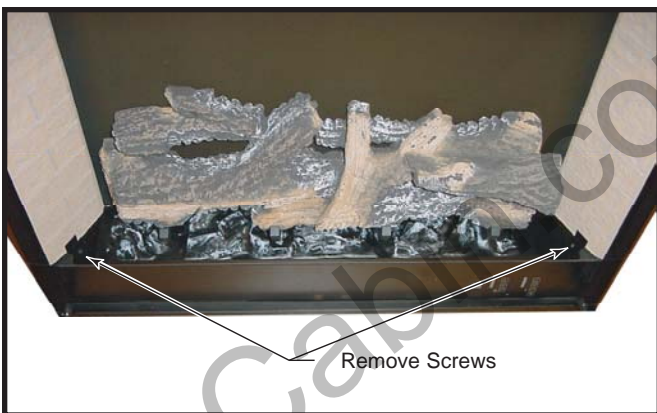
Fig. 6 Remove screws that hold refractory bracket with ember bed.
