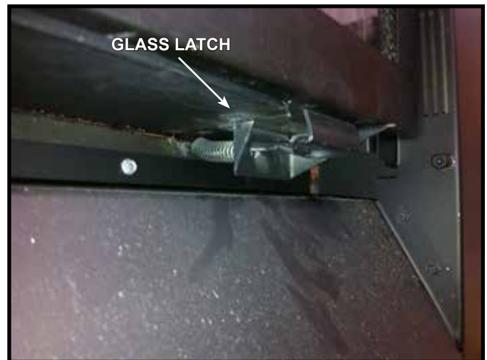
4.4 Glass Latch Detail - Exterior Side
