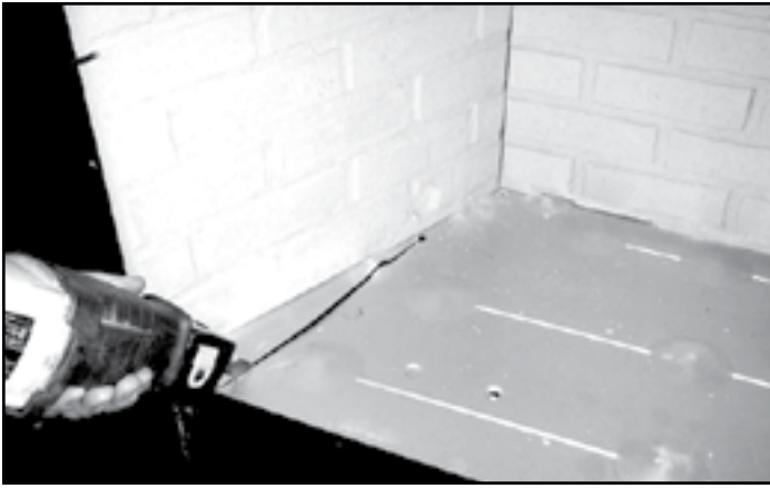
Figure 12.1 - Using a saws-all, cut out the floor.
