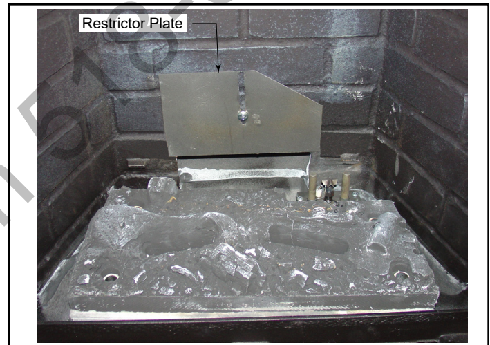
Figure 9 - Loosen screw to adjust restrictor plate.
