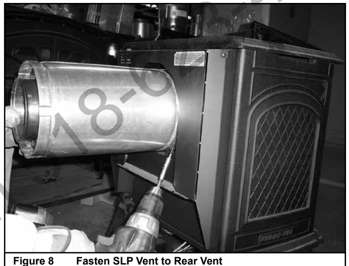
Figure 8 Fasten SLP Vent to Rear Vent
