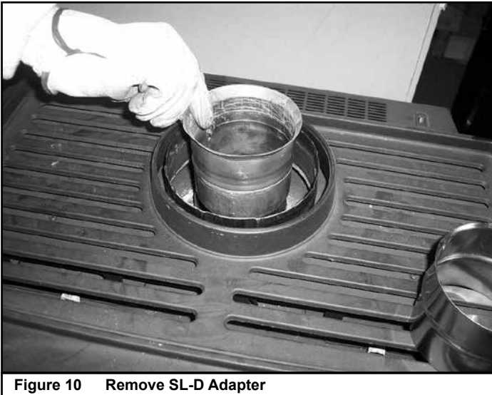
Figure 10 Remove SL-D Adapter
