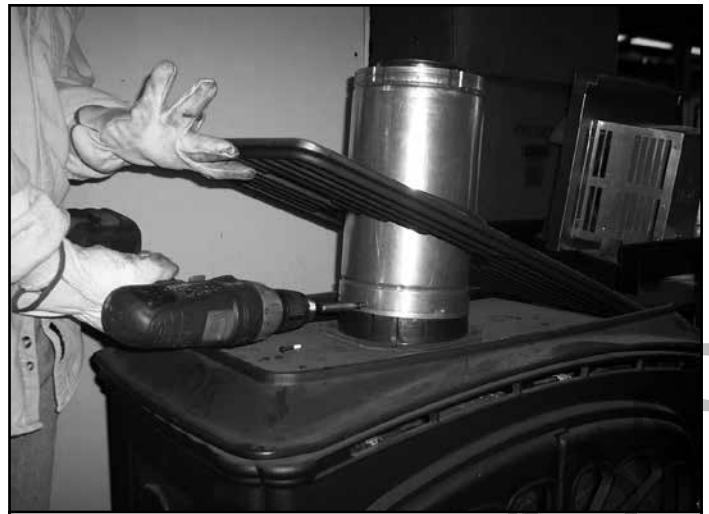
Figure 7 Fasten SLP Vent to Stove
