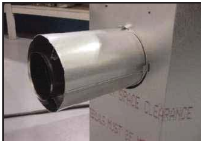
Figure 7.10 Attach the first vent section (it will snap into place). Slide the insulation gasket onto the vent section, up against the appliance and over the tabs.
