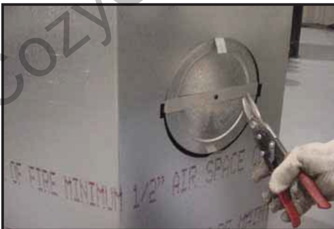
Figure 7.7 Cut the metal retaining band and fold the sides out.
