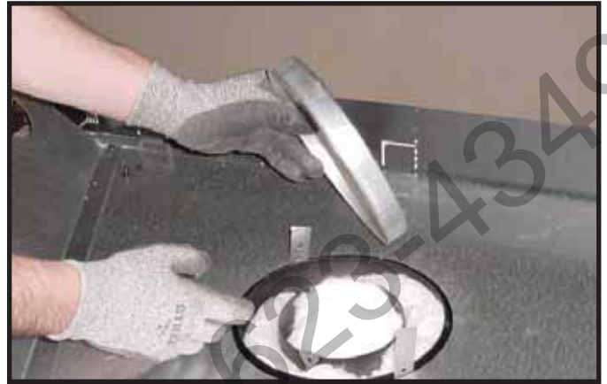
Figure 7.4 Remove the seal cap.
