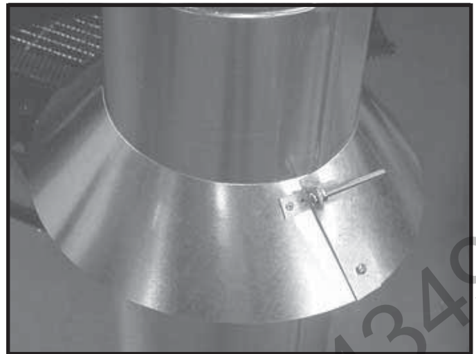
Figure 8.20 Assembling the Storm Collar Around the Pipe
