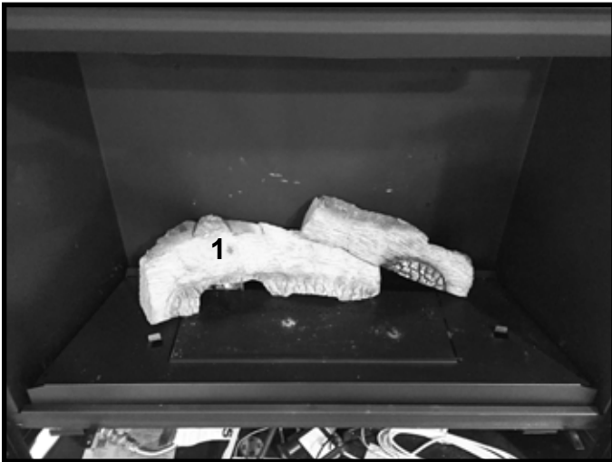
Figure 4. Install Left Rear Base Log
