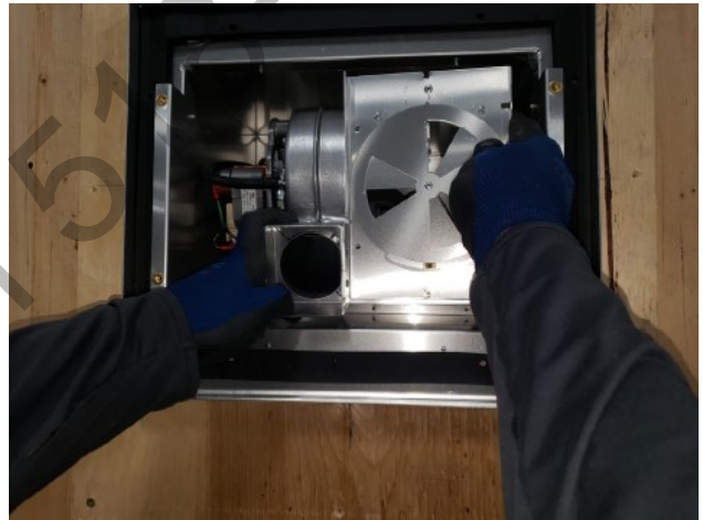
Figure 8.3 - Exhaust Assembly Removal
