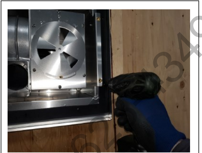
Figure 6.6 - Secure Power Vent to Exterior
