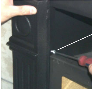
Secure top of faceplate with screw.
