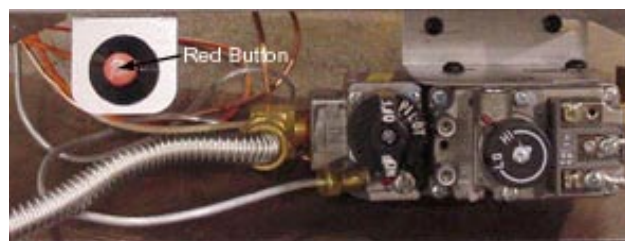
Figure 24 - Standing Pilot Ignition
