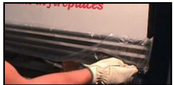
Figure 20 - Control Access Panel Removal
