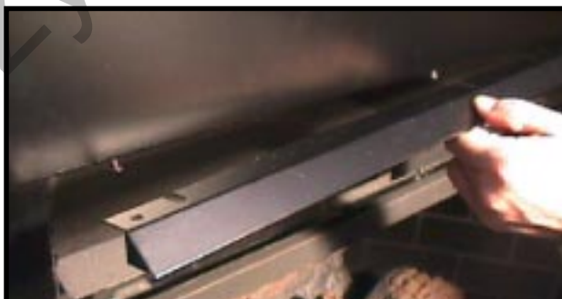
Figure 18 - Hood Placement
