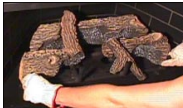
Figure 32 - Log Removal (33-36 Log Set Shown)
