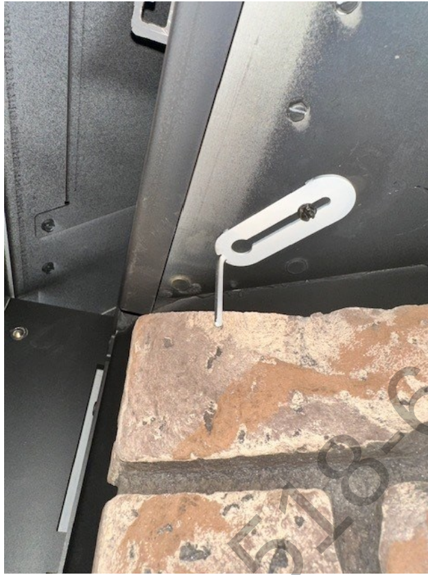
Figure 5 - Side Refractory - Panel Clip Location & Installation
