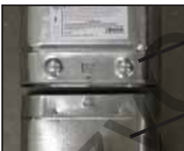
Illustration 2 - Adding Selkirk Model OV Oval Gas Vent
