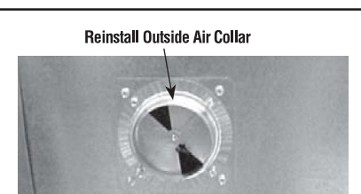
Figure 14 - Reinstall Connector
