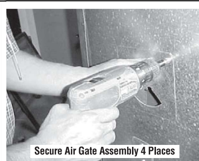
Figure 13 - Install Screws
