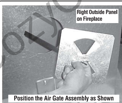
Figure 10 - Air Gate Assembly to Fireplace
