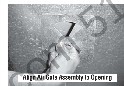
Figure 12 - Position Air Gate
