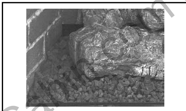
Figure 44 - Installing the volcanic stone
