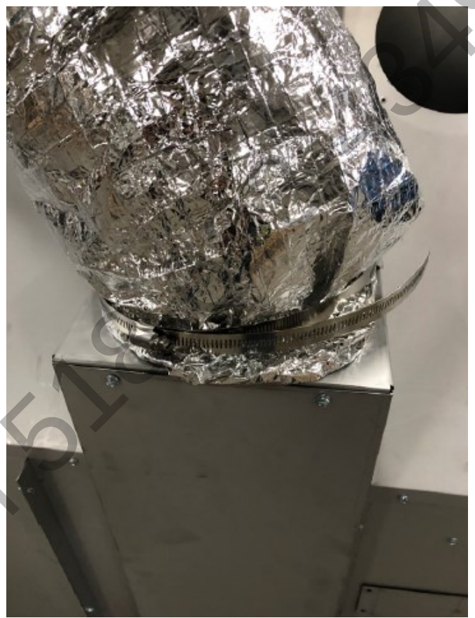
Figure 2.4, Band clamp securing insulation
