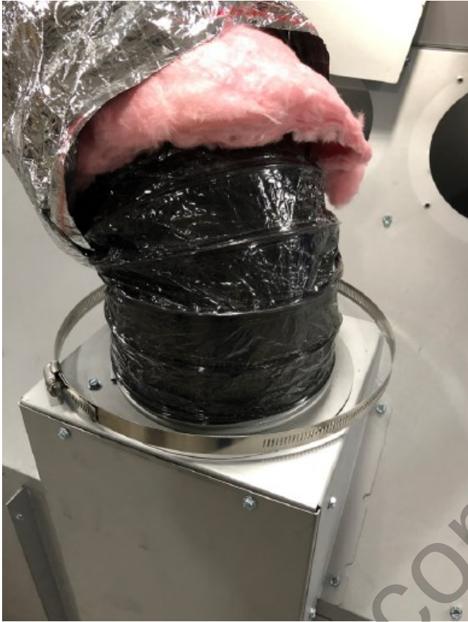
Figure 2.3, Attach Inner duct
