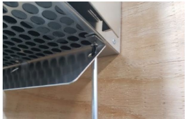
Figure 2.16 - Vinyl Siding Shield Installed
