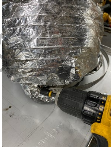
Figure 2.15 - Install Outer Liner with Band Clamp
