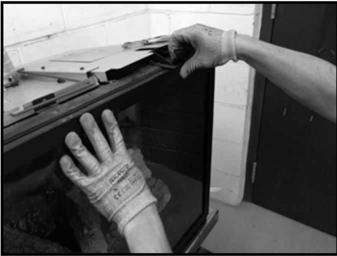
Figure 11.4 Release Glass Latches One at a Time
