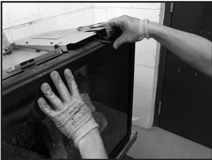
Figure 4.3 Release Glass Latches One at a Time
