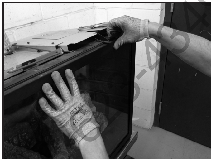
Figure 11.3 Release Glass Latches One at a Time
