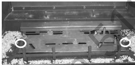
Remove 2 screws, then push burner tray to left and lift out.
