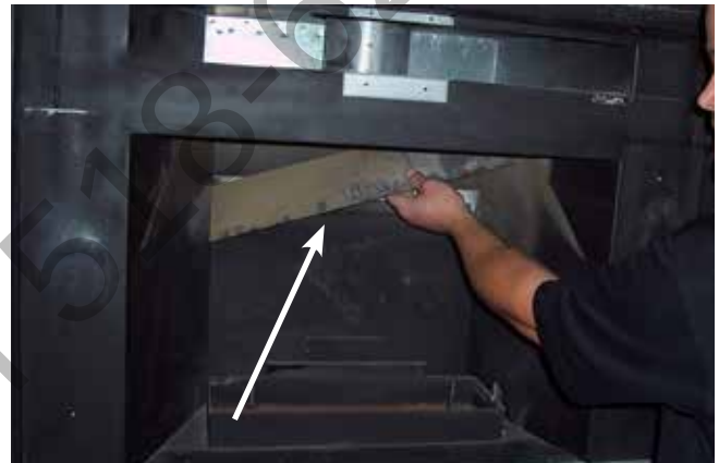
Remove rear baffle
