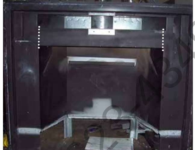
Cut out front cross piece to remove
