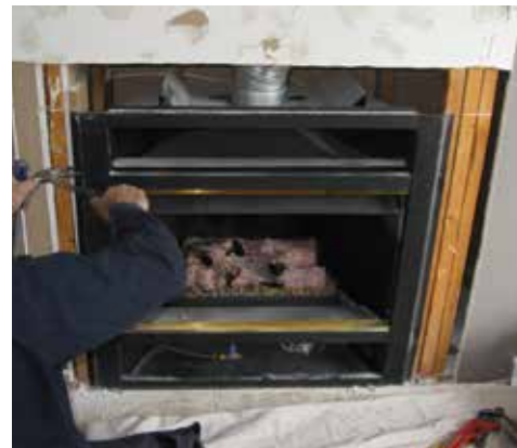
Remove unit from framing
