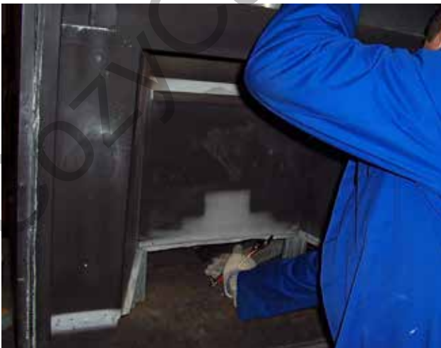
Flatten louver brackets
