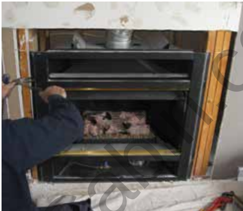
Remove unit from framing
