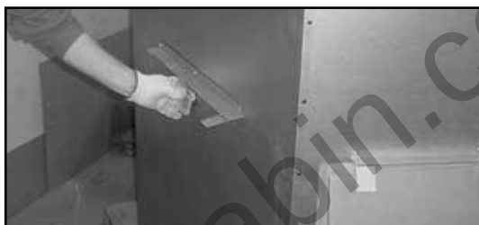
Figure 3.7 Bending Refractory Shipping Tabs Back Down
