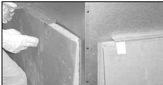
Figure 3.6 Unpacking Back Refractory
