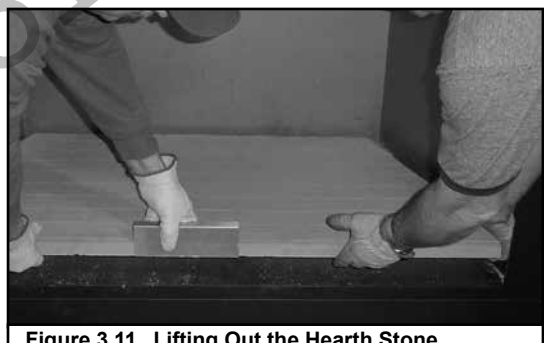
Figure 3.11 Lifting Out the Hearth Stone
