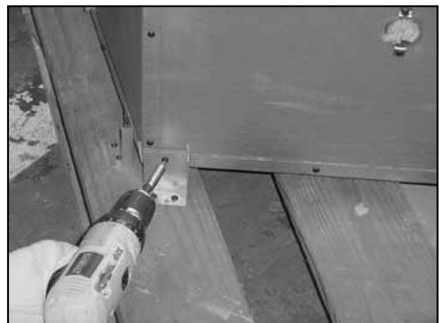
Figure 3.12 Removing Shipping Brackets
