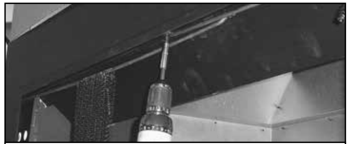
Figure 3.9 Removing the Screen Rods
