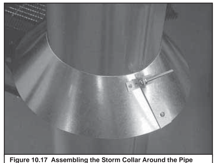
Figure 10.16 Assembling the Storm Collar
