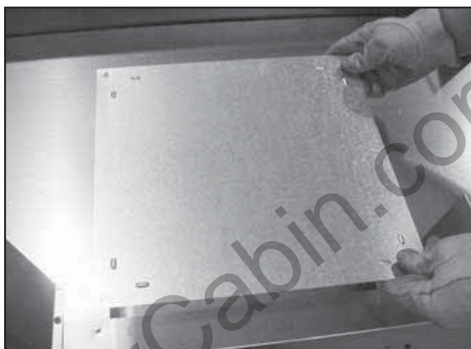
Figure 9.17 Place Cover Plate on Top of Appliance
