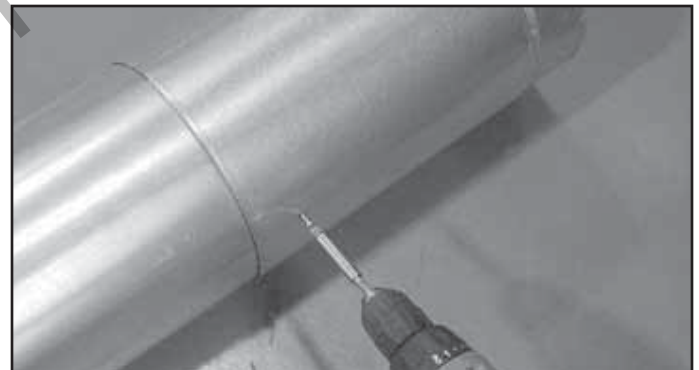
Figure 10.7 Screws into Slip Section
