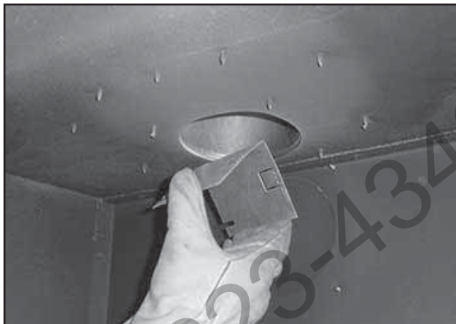
Figure 7.19 Placing the Baffle
