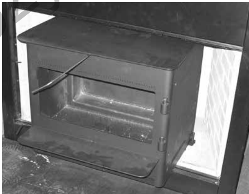
Diagram 5: Pull Rod In Place
