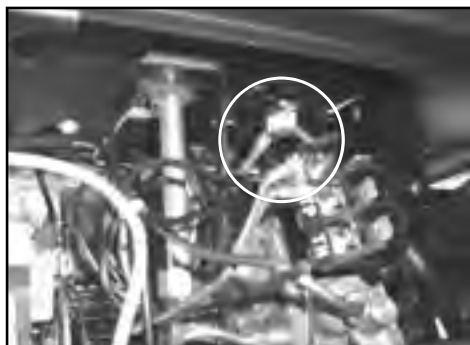
Figure 43: Installing Temperature Sensor.
