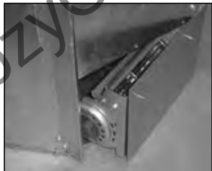
Figure 48: Installing Fan Through the Back.
