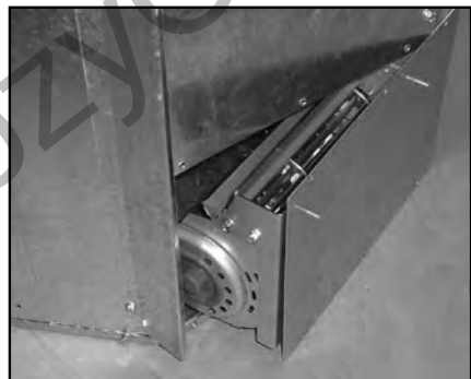
Figure 48: Installing Fan Through the Back.
