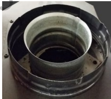
Vent Attachment Inspection – unbent and attached rings
