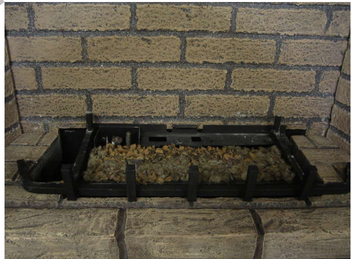
Figure 50 - Rock wool placement
