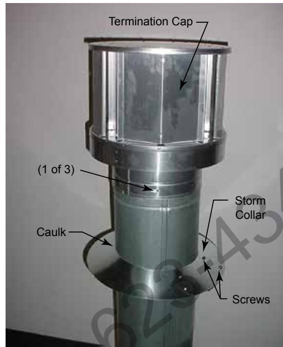
Figure 63 – Secure with Screws
