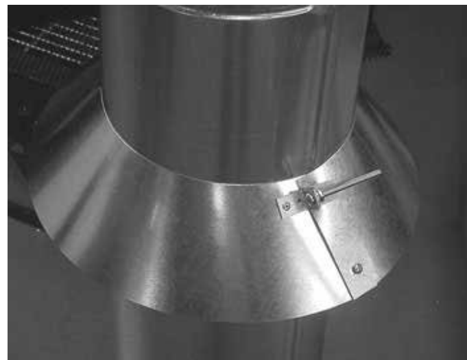
Figure 62 – Insert Bolt into Brackets
