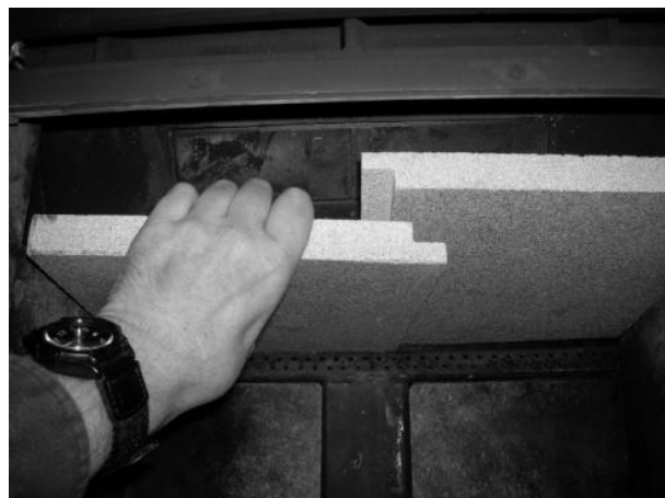
Figure 16 - Removing/Replacing the Baffle for Inspection
