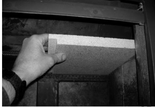
Figure 16 (cont.) - Removing/Replacing the Baffle for Inspection
