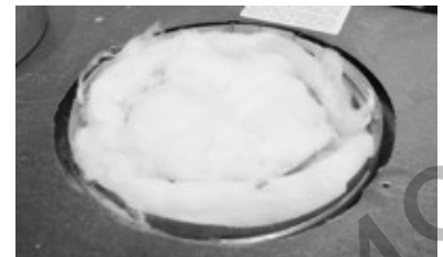
Step 3: Remove insulation from inside flue pipe.
