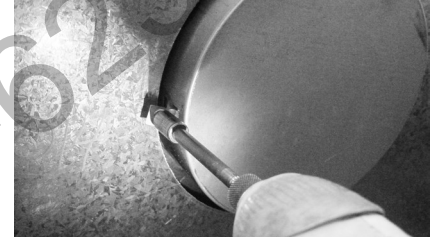
Step 5: Bend tabs out on round flue cover. Secure the round flue cover (provided) to the wrapper over the rear venting outlet. Use two (2) 3/4" long sheet metal screws
