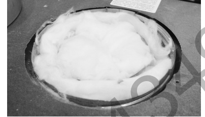
Step 3: Remove insulation from inside flue pipe.
