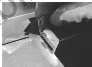
Step 1: Carefully bend up the two (2) tabs on the heat shield at a 90° angle from each opposite joint and then the foot of the Standoff at approximately a 45° angle.
