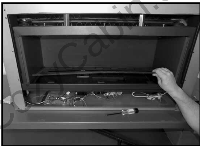
Figure 45: Inserting glass media tray.
