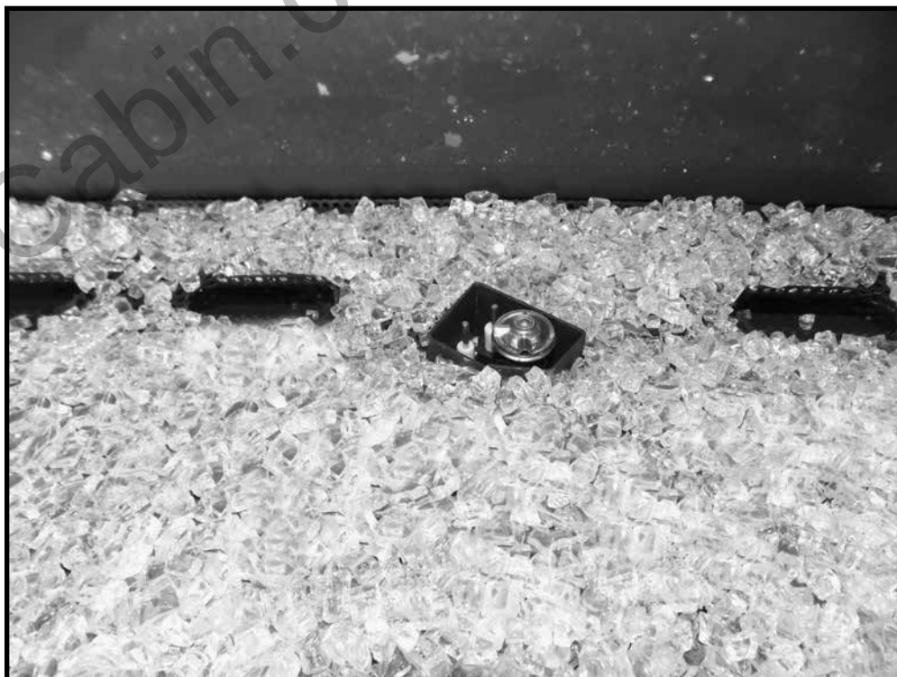
Figure 53: Glass media installation.
